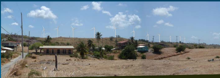
VIEW OF THE LAMBERTS EAST WIND FARM FROM RISK ROAD
