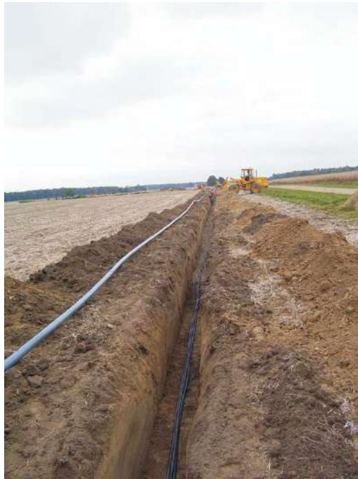
LAYING UNDERGROUND POWER CABLE
